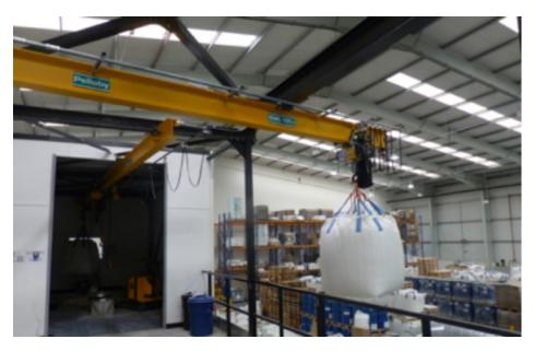
One tonne bags of silicone are regularly transported to a mezzanine floor within Multisorb's large warehouse in order to be loaded from above into special equipment for further processing. Until recently these bags were lifted to the mezzanine level via a forklift truck and a goods lift, before finally being taken to the station via two existing Pelloby post mounted monorail cranes.
