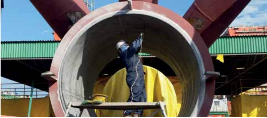
Above: Belzona bonding application for riser bearings and caissons
