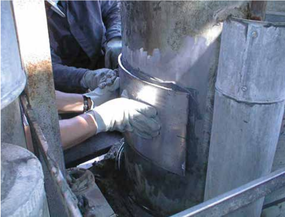
Above: Picture 1: Plate bonding repair on equipment
