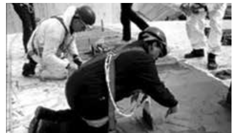
Above: Picture 5-6: Application on site.
