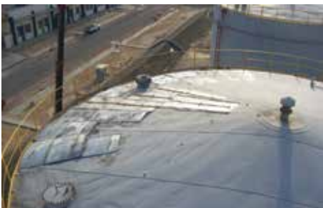
Above: Picture 2- 3: Storage tank roof repaired using Belzona
