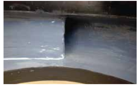
Above: Pump cutwater rebuilt and protected against abrasion and high temperature
