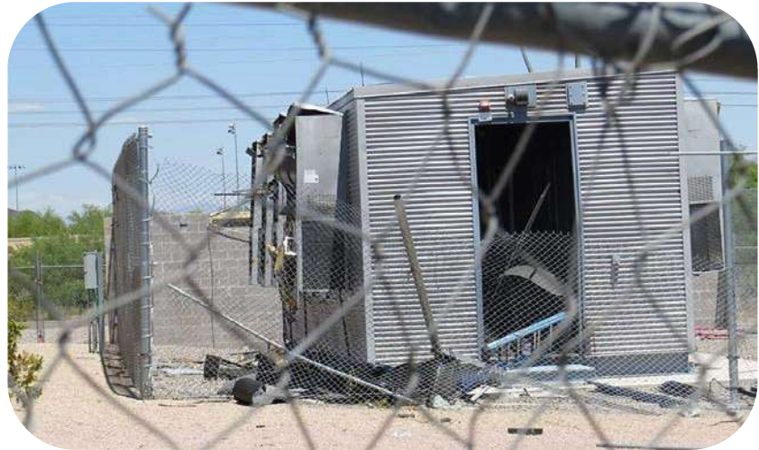
Fig. 1 + 2: Damage to a battery energy storage system after an explosion, Arizona Public Service, 2020 ( https://spectrum.ieee.org/dispute-erupts-over-what-sparked-an-explosive-liion-energy-storage-accident , 11.11.2021)
